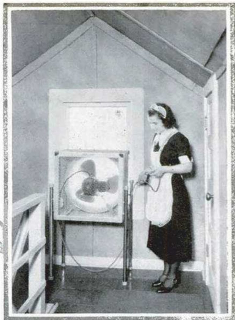
AIR PURIFIER. This air circulator is installed in the attic of a house and electrically operated. It has a three-blade fan that causes a steady circulation of air so odors and smoke are drawn from the lower rooms
